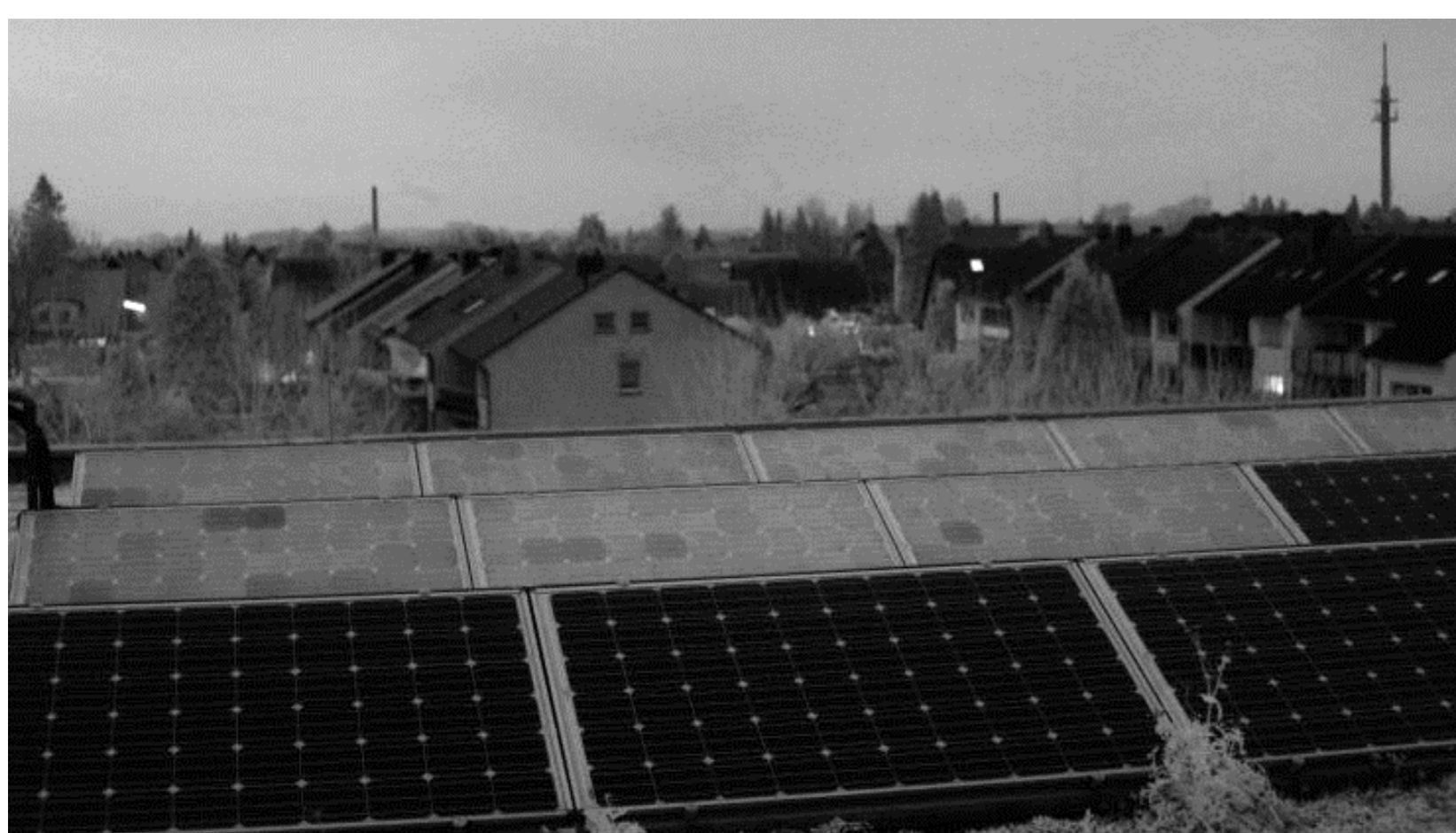
Fig. 7: EL exposure with extraneous light at dawn with reverse current feeding of the rear modules
